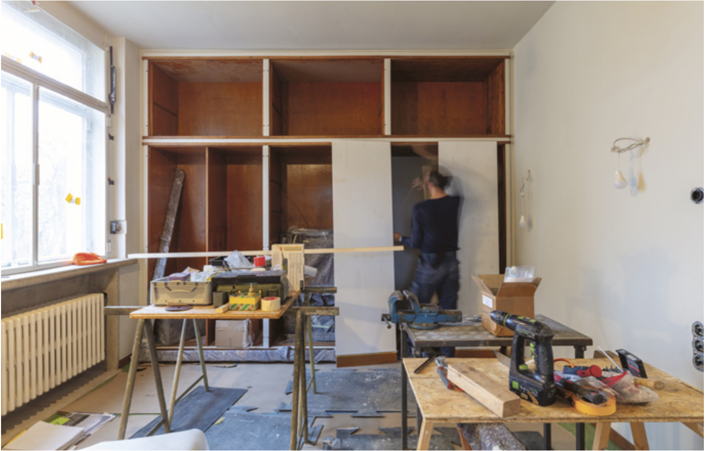
The 16 built-in cupboards were restored both on- and off-site, and missing parts were replaced.
