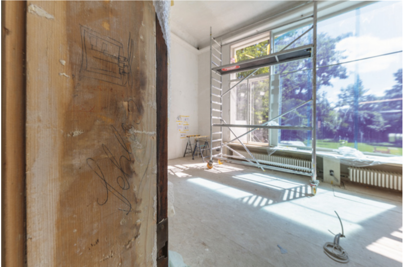
Labels and electrical wiring diagram from the original construction on the door frame to the dining room.
