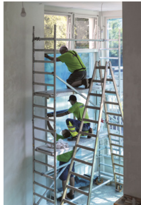
Applying protective film to the new windowpanes.
