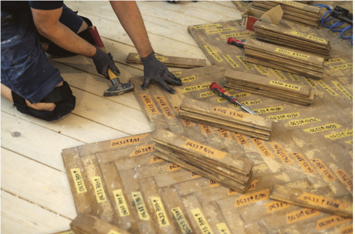
More than 5,000 parquet strips were removed and, after refurbishing the subfloor, reinstalled in their original pattern.
