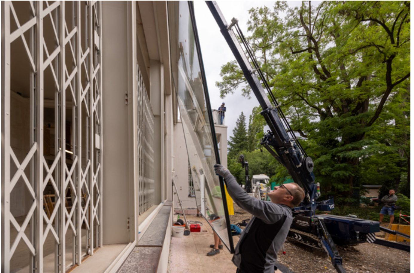
Installation of the large insulating glass pane in the dining room.
