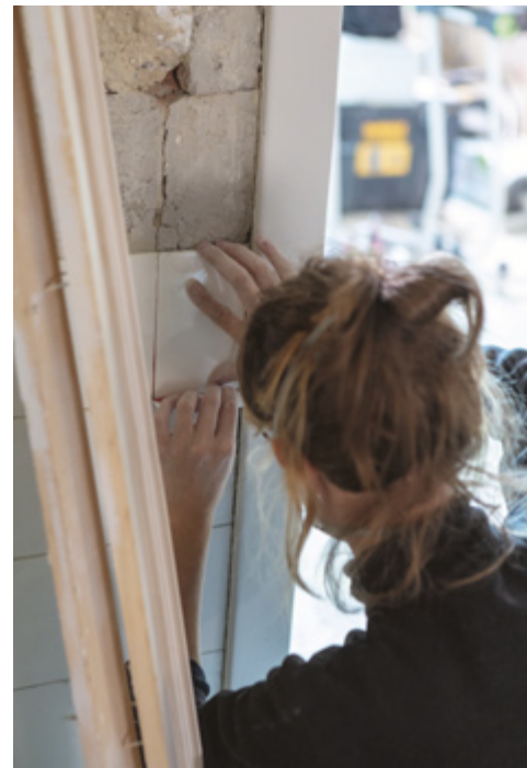
Replacing missing bathroom tiles with historical finds.
